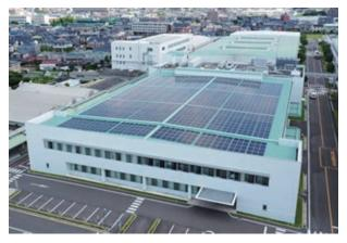
As an initiative for incorporating renewable energy design, in July 2020 we installed and began operation of a solar power generation system at the CKD Head Office/Komaki Plant. It is expected to reduce annual CO<sub>2</sub> emissions by 300 tons. Going forward, we plan to systematically install these systems at our other plants in Japan and overseas.
